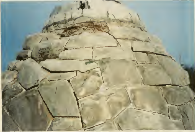
Figure 19: Green paint on the rock mound base (Photograph by author, March 2002)
